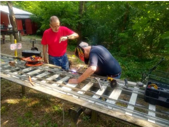
Ed observing while Carl welds in a replacement rail after a tree limb damaged the unloader track.
