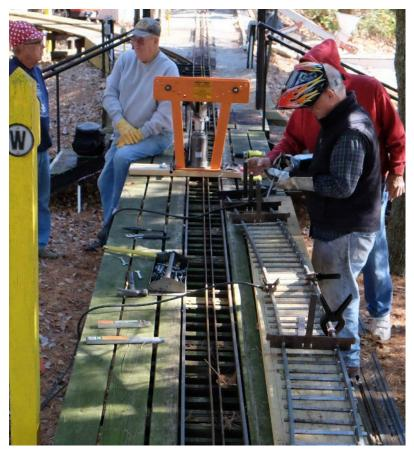
The second (inside) rail is then added using gauges to ensure 7%" spacing for 1%" scale rolling stock. Likewise, middle rails are added for 3/4" and 1" scale.
