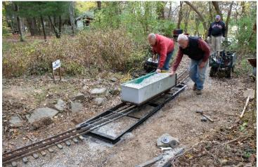
Oct 22: The Test: A section of the main line was cut out and in its place a "frame" upon which a "flexible track section" rests, both built by Carl Schwab, was installed in its place. Like all other turnouts on the property, the flex-track will serve as "switch points" when the turnout is completed.
