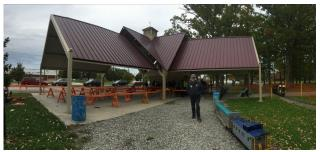
They have 2 train sheds—tube-like—to store the locomotive and cars assigned to this location. There are 2 loader tracks, one fixed (most likely the original loader), and one like a transfer table. Neither adjust vertically, although they have long bridges.
