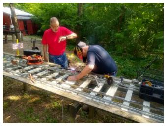
Ed observing while Carl welds in a replacement rail after a tree limb damaged the unloader track.
