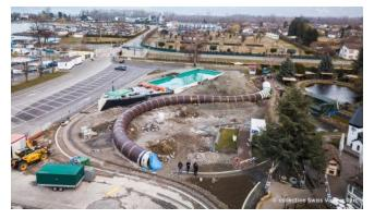
Four acres of 7.25" gage steam, miniature buildings, and artificial mountains, meticulously landscaped. Here is an expansion they have been doing. Since they are landlocked, they built a huge concrete underground car barn and serpentine tunnel from prefabbed concrete sections
