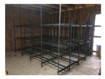
Checked for square and level again, then attached some  $1'' \times 1/8''$  cross-brace strapping along the back.
